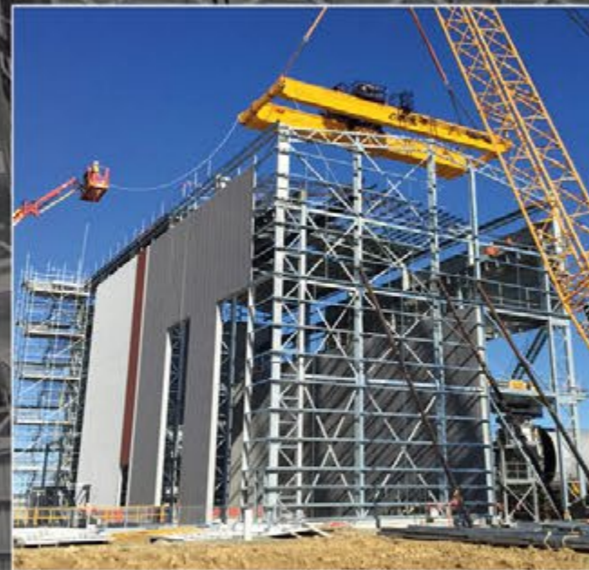
Crane installation at Veolia site
