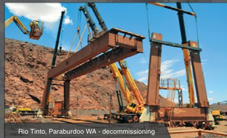
and installation of the 80/16t x 34.1m FPZLK primary crusher crane
